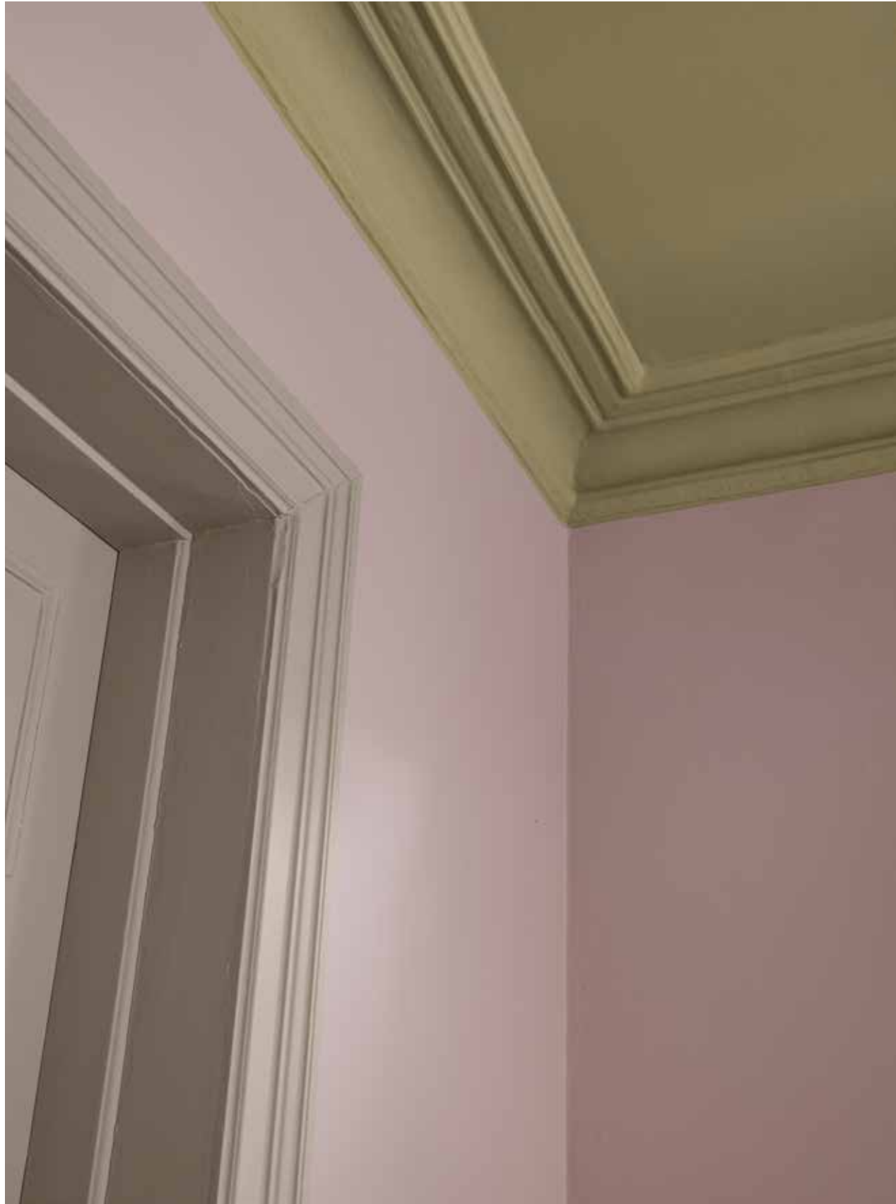
Wall: Paint Desert Rose Ceiling: Old Yellow Bloke Wooden Door: Paint Life Is A Rose Floor: Paint Tangled Up
