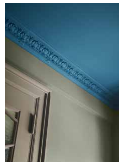
Wall: Green & Gold Wooden Door: Paint Life Is A Rose Ceiling: Paint Sweet Peas Floor: Paint Tangled Up Wall: Green & Gold Wooden Door: Paint Paint Life Is A Rose Ceiling: Dolphins Opposite Page, Wall: Paint Blue In Green, Nights In White Silk, Tangled Up and Castle Made Of Sand Wooden Door: Paint Sweet Peas
