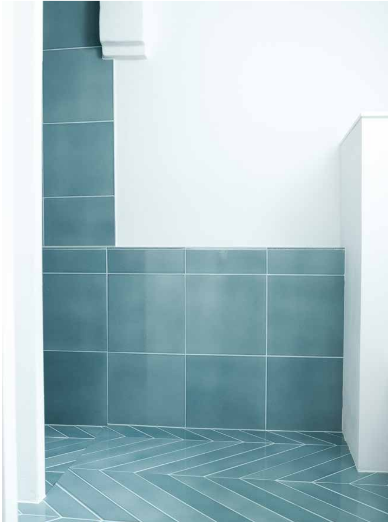
Wall: Paint White Tail Wall: Tile Bespoke Format Lava Stone Shiny Crystal / Blue Smoke Floor: Tile Bespoke Chevron Lava Stone Shiny Crystal / Blue Smoke
